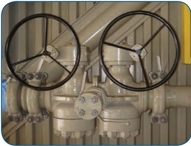
The valves illustrated are 6" class 2500 with hub ends, in carbon steel, manually operated. Criteria for selection: bubble tight isolation and compact design.
