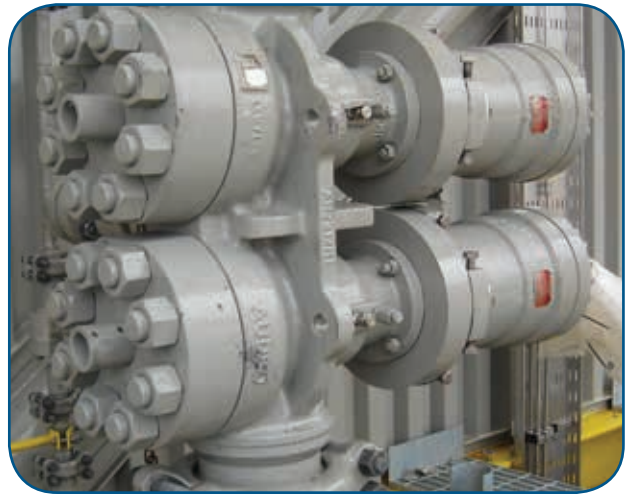
The valves illustrated are 12" class 2500 with hub ends. Criteria for selection: tight shut off, safety reliability and low maintenance.
