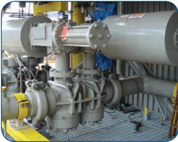
The valves illustrated are 12" class 2500 with hub ends. Criteria for selection: tight shut off, safety reliability and low maintenance.
