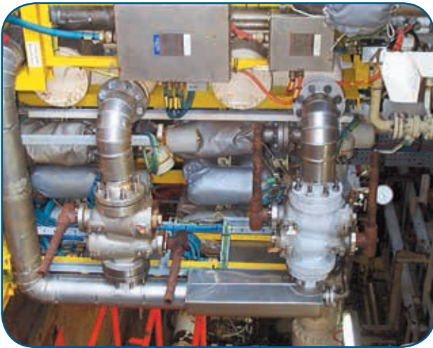
The valves illustrated are 4" class 300 flanged in Carbon Steel and Stainless Steel. The application is on a fuel skid and both plugs on each valve are lever operated. Criteria for selection: double block and bleed with true bubble tight isolation for reasons of safety, reliability and minimum maintenance.
