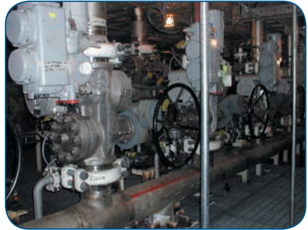
The valves illustrated are 8" class 1500 Double Isolation Plug Valves in 25% Cr. Duplex with hub ends. The valves are installed on a flowline header application. In this case one isolation is by electric actuator and the other isolation is by gear operator. Criteria for selection: true bubble tight isolation and space and weight saving over conventional ball or gate valves and minimum maintenance.
